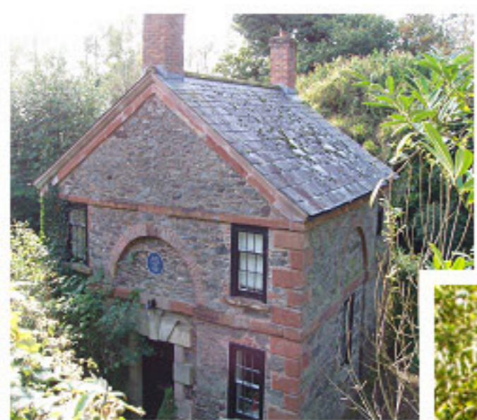
Lock Keeper's House Lock No 6
